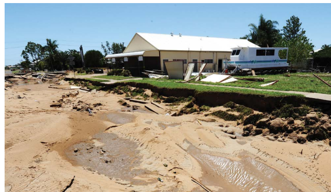
Bundaberg, Queensland February 2013
